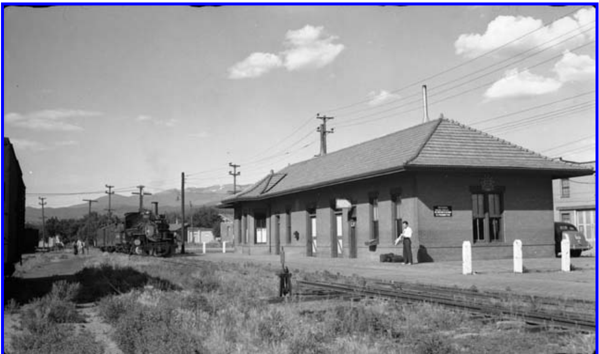
Old Santa Fe Depot
